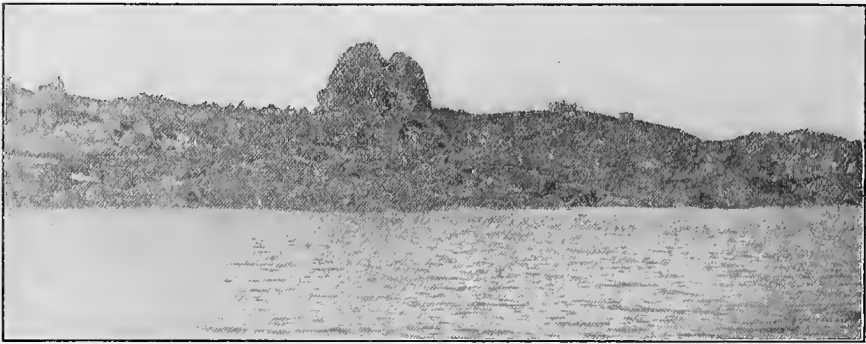
THE ROCK OF KONOSSO IN JANUARY, 1902, BEFORE THE BUILDING OF THE DAM AND FORMATION OF THE RESERVOIR.
